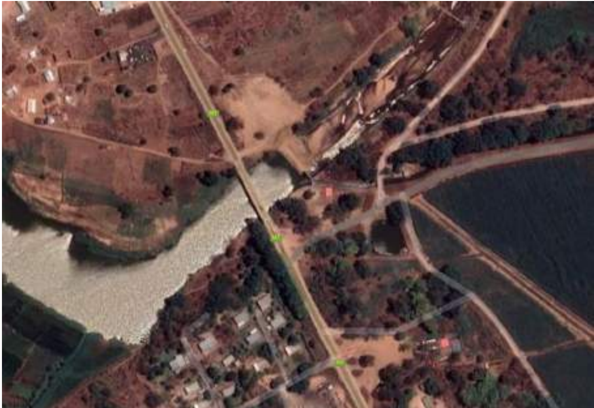
FIGURE 6-2: Weir downstream the Dwangwa Bridge
