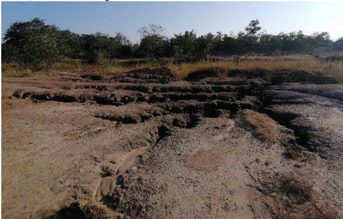
Plate 5-12: Erosion in the southern site into the southern river looking onto the sand mine.
